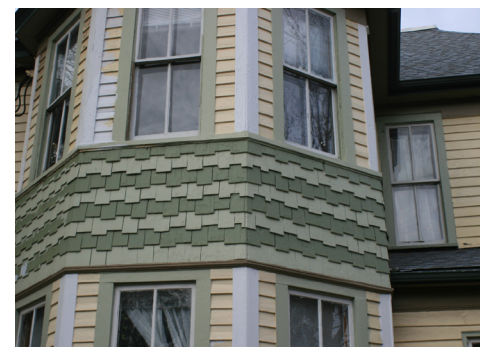
Wood siding provides texture and allows for contours that cannot be replicated with synthetic sidings.
