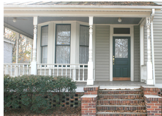
These simple, unobtrusive light fixtures are mounted to the porch ceiling.
