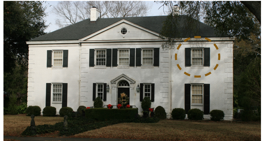
Shutters fit the window opening and are in keeping with the architectural style.
