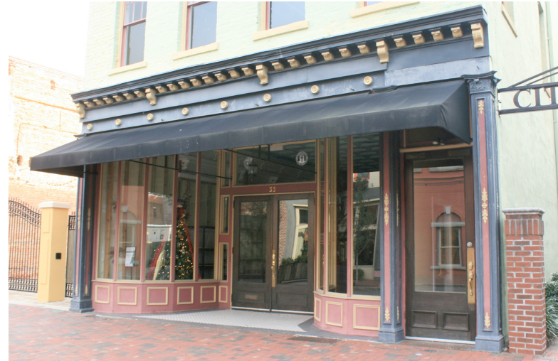
The recessed entrance and storefront cornice are character-defining features of this commercial building.
