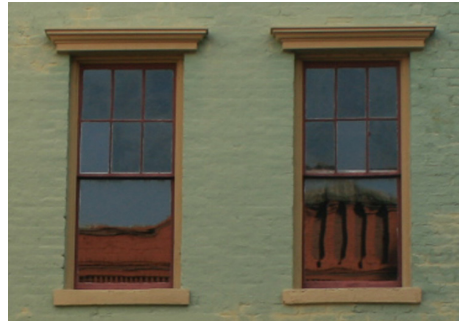
Double-Hung Sash with Decorative Lintel
