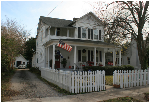
This low fence with painted wood pickets coordinates with the color and materials of the house.
