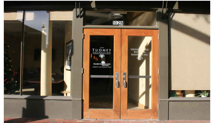
These appropriate wood replacement doors are single light.
