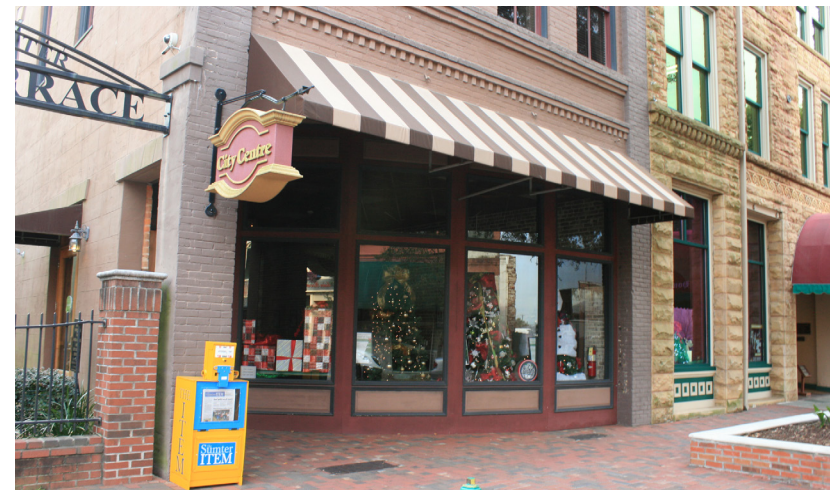
The transom and bulkheads of this storefront are simple in design and are based on the scale, proportions, materials and colors of other commercial buildings in the district.
