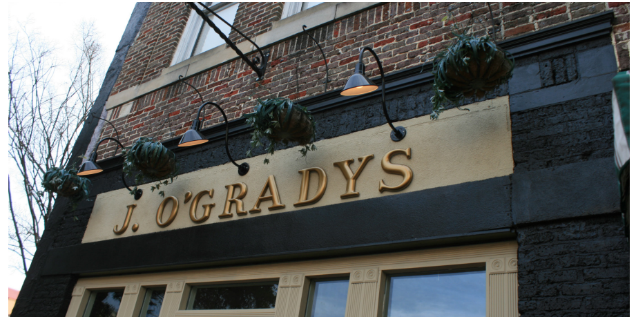
Sign illuminated indirectly with shielded light source.
