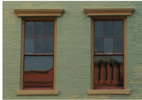
Double-Hung Sash with Decorative Lintel
