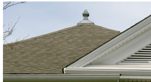
Reinstalled finial after roof replacement.
