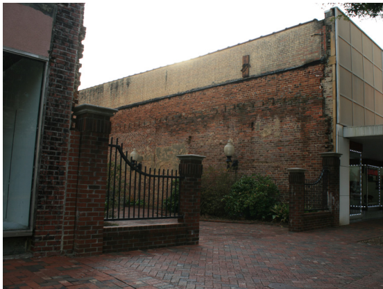
The brick piers continue the street wall while the open metal pickets allow views to the courtyard beyond.
