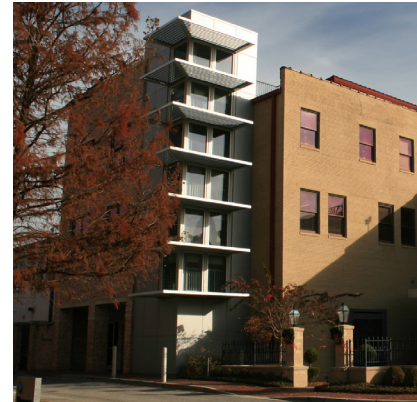
Located on the rear elevation, this addition is contemporary in design to distinguish it from the original building.
