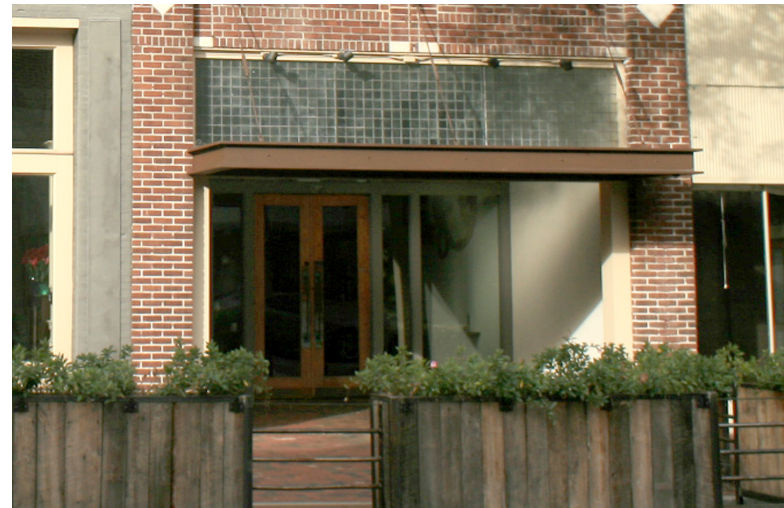
Preserve original transom materials, such as prism glass.
