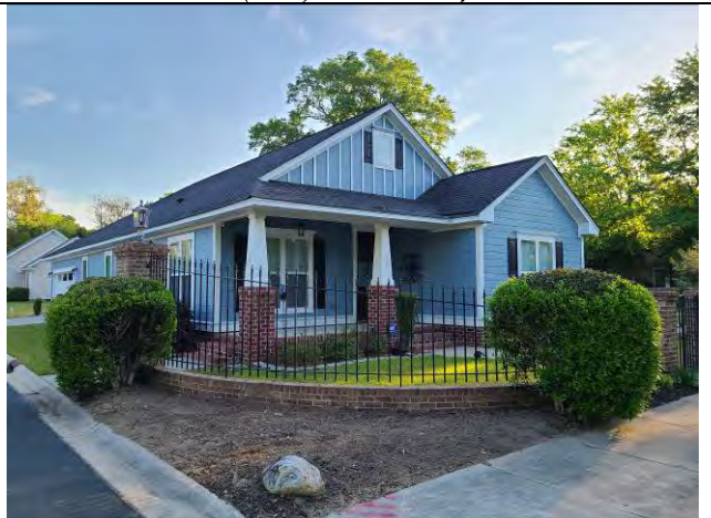
Existing residence at 10 Calhoun Pl.
